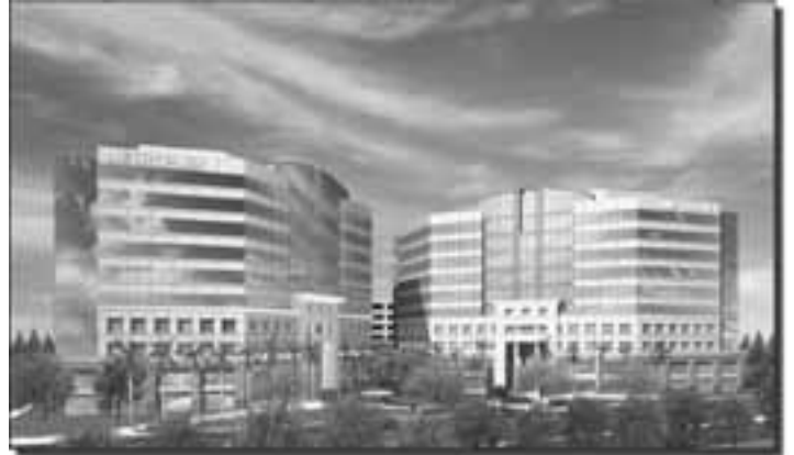
The first tower of the Metroplex Office Center, under construction at 1401 Willow Pass Rd., is slated for completion in 2002.
