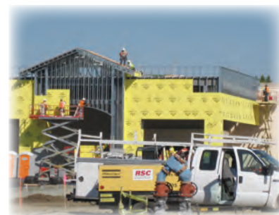
Lowe's Shopping Center under construction
